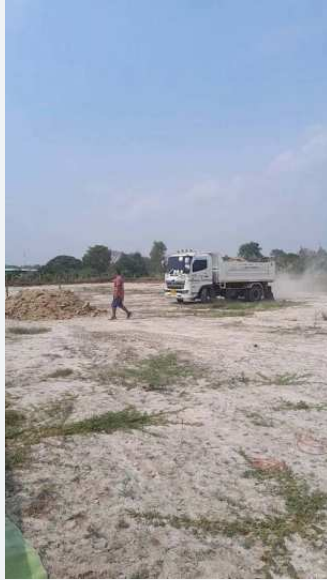
Site grading and early ground-preparation activities.
