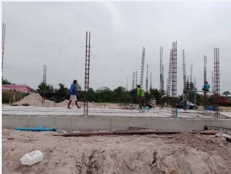
Work in progress around reinforced concrete elements.
