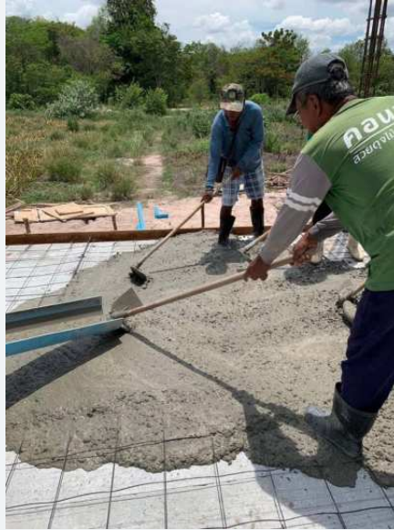
Concrete placement at the building site.
