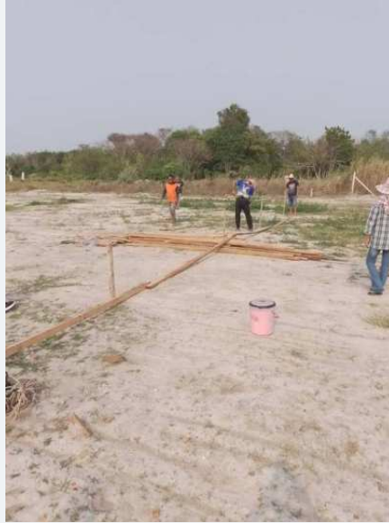
Site setting-out and surface preparation.
