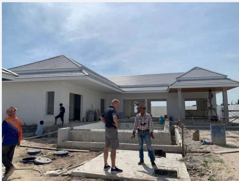
Site photograph showing the evolving building form.
