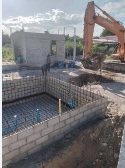
Wall construction around the structural frame.
