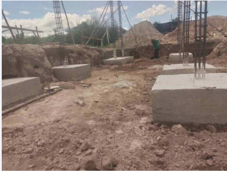
Excavation and foundation preparation in progress.
