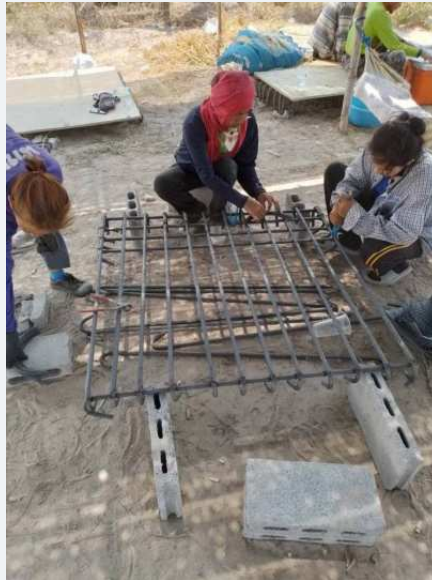
Placement and arrangement of reinforcing steel.
