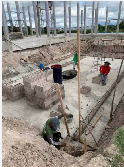
Masonry wall construction and building enclosure.
