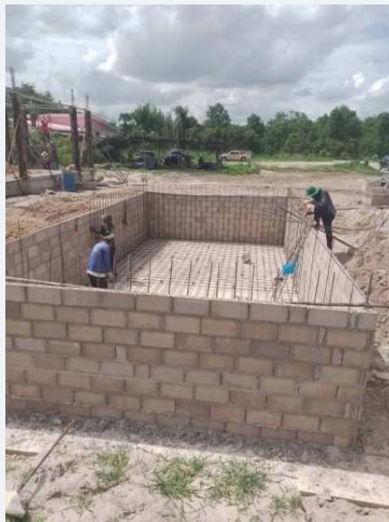
Progress of blockwork and external wall formation.
