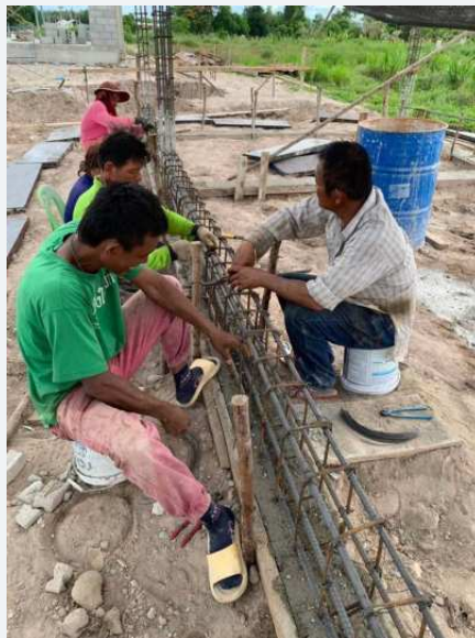
Placement and arrangement of reinforcing steel.
