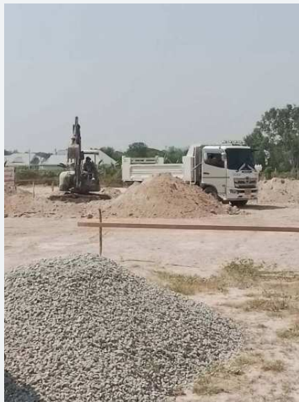
Site setting-out and surface preparation.
