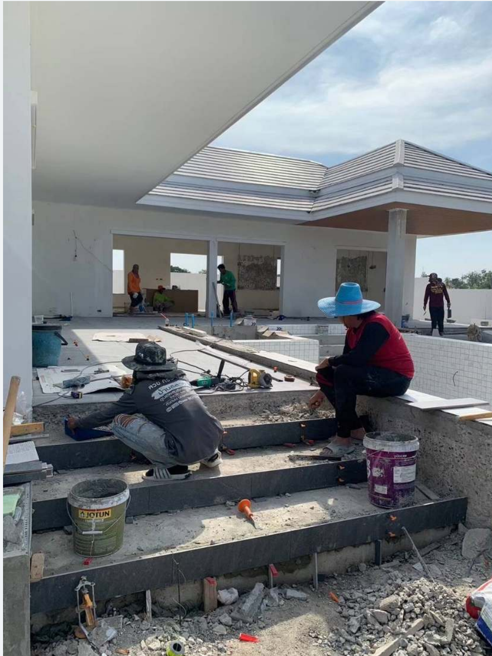
Overall view of the building during construction.
