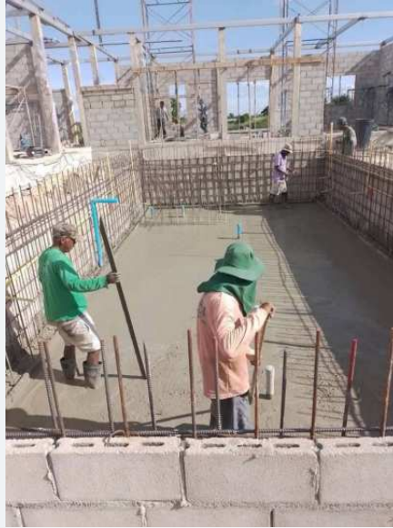
Slab formation and concrete finishing activities.
