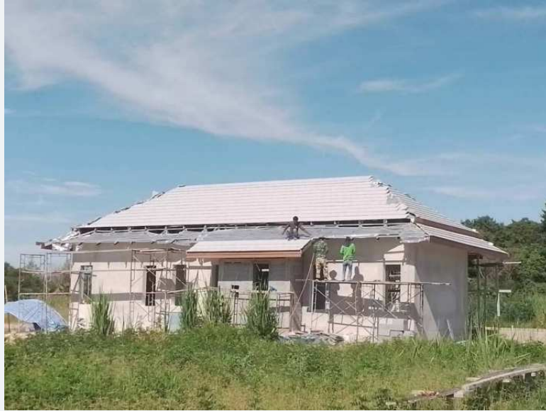
Work progress viewed from the surrounding site.
