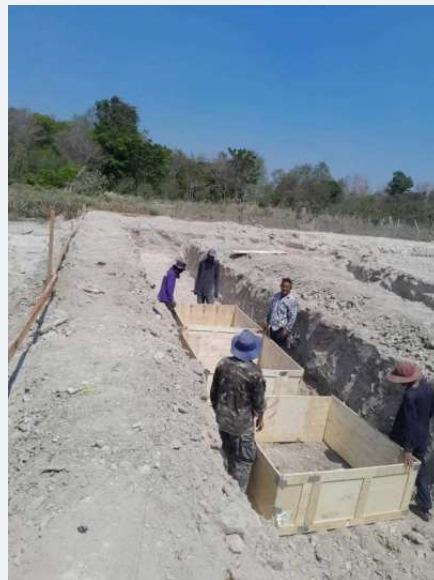
Concrete footings and associated foundation work.
