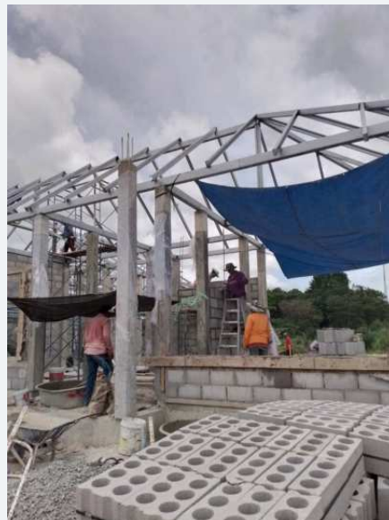
Building-services installation and finishing-stage activities.
