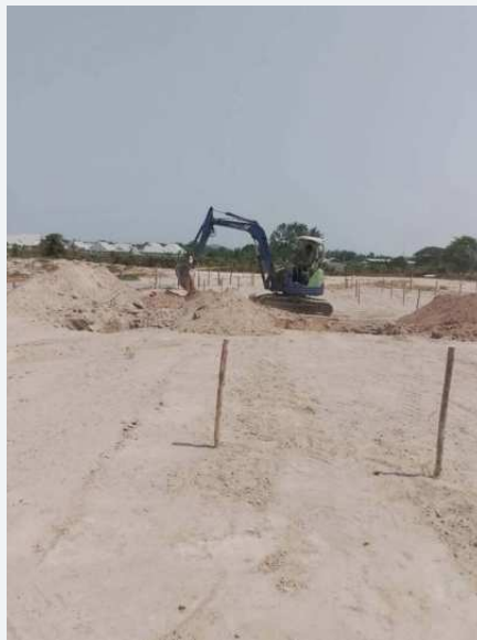
Earthwork and construction-area preparation.
