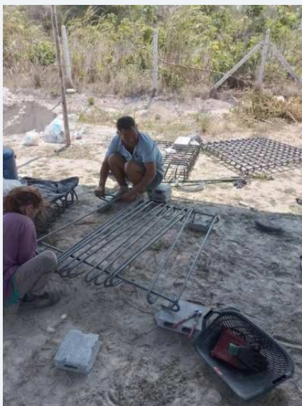
Steel reinforcement before subsequent concrete works.
