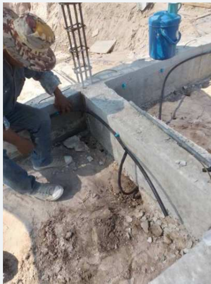
Preparatory work around the structural foundation area.
