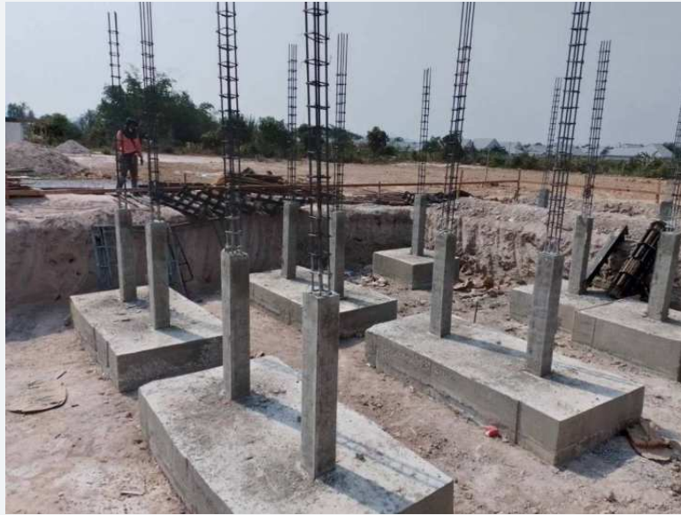
Structural frame works during the construction stage.
