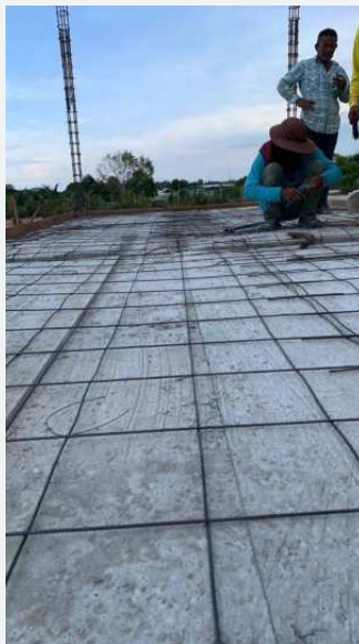
Reinforcement detailing and formwork preparation.
