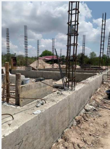
Steel reinforcement before subsequent concrete works.
