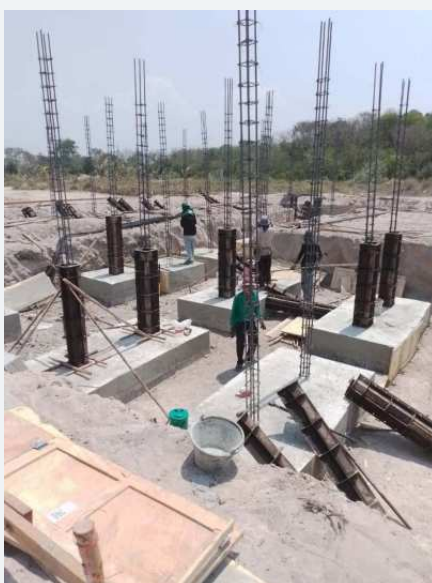
Placement and arrangement of reinforcing steel.
