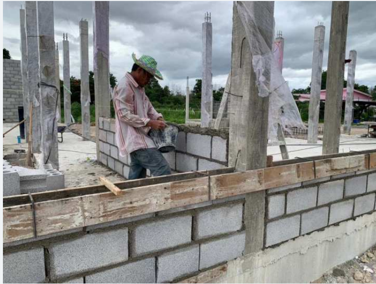
Progress of blockwork and external wall formation.
