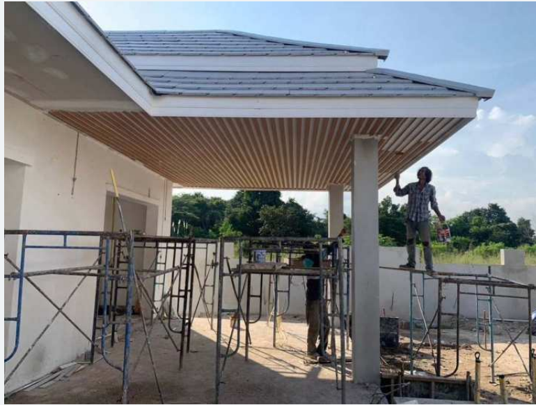
Overall view of the building during construction.
