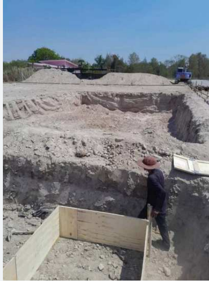
Concrete footings and associated foundation work.
