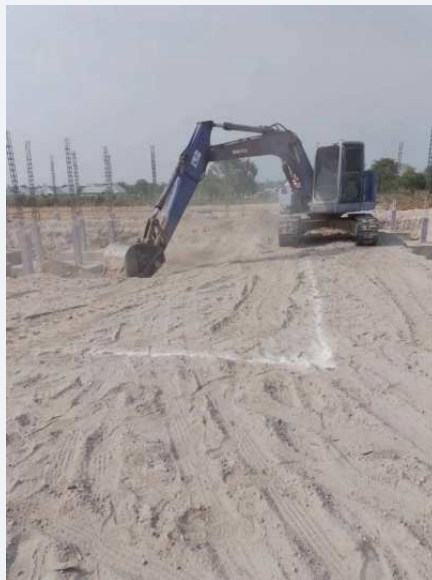
Site grading and early ground-preparation activities.
