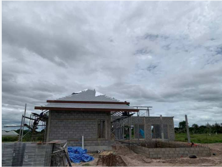
Site photograph showing the evolving building form.
