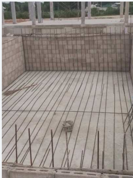
Steel reinforcement before subsequent concrete works.
