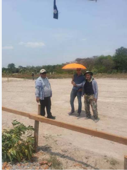
Earthwork and construction-area preparation.
