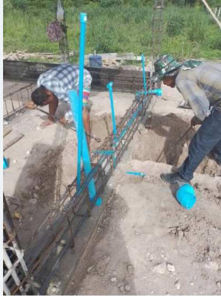
Concrete footings and associated foundation work.
