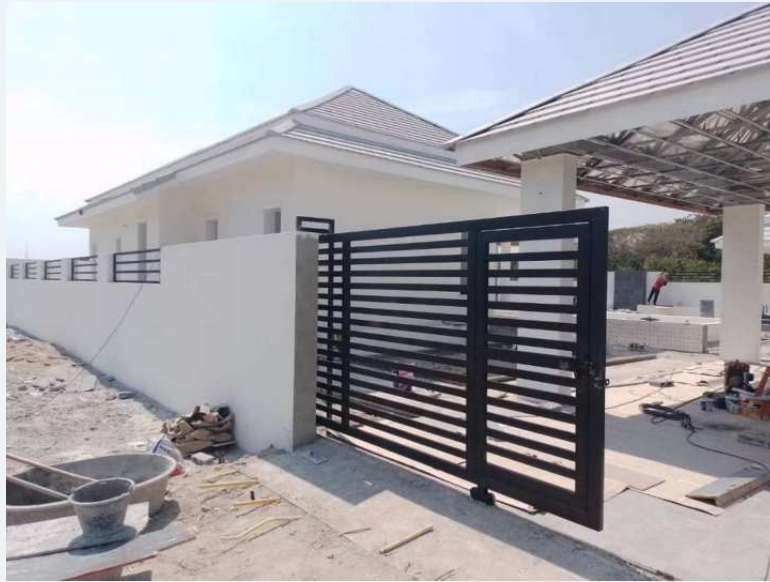
Work progress viewed from the surrounding site.
