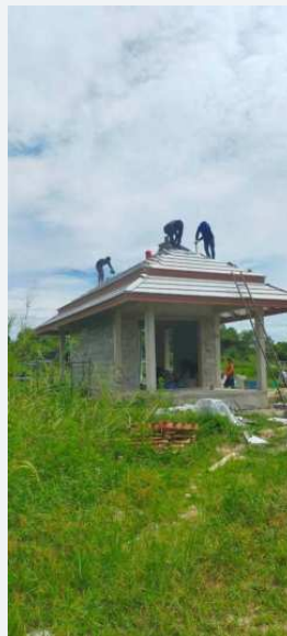
Site photograph showing the evolving building form.
