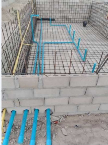
Masonry wall construction and building enclosure.
