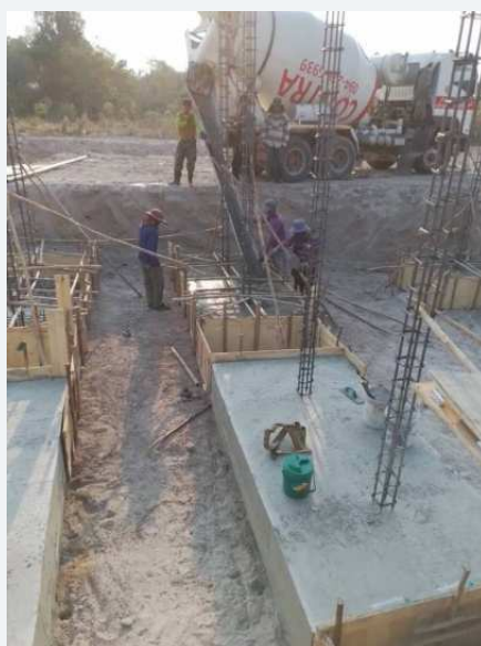
Reinforcement detailing and formwork preparation.
