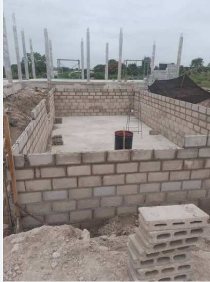
Masonry wall construction and building enclosure.
