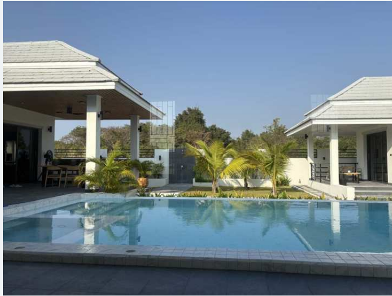
Pool-facing outdoor living area and residential building frontage.
