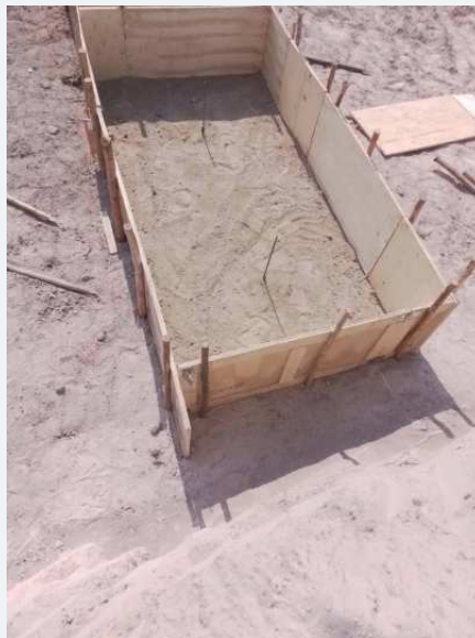
Preparatory work around the structural foundation area.
