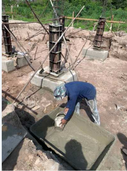
Concrete placement at the building site.
