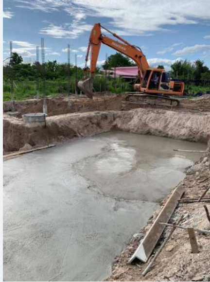
Site grading and early ground-preparation activities.
