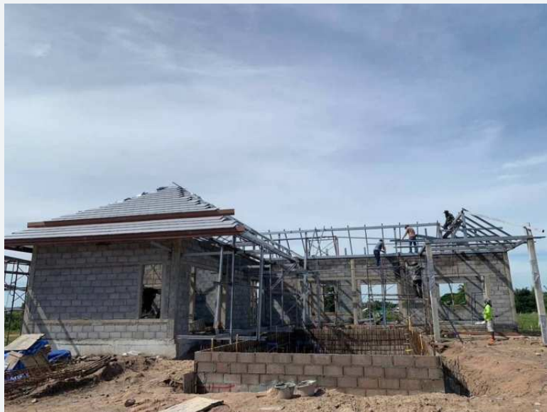
Work progress viewed from the surrounding site.
