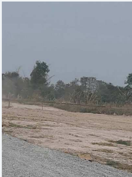
Earthwork and construction-area preparation.
