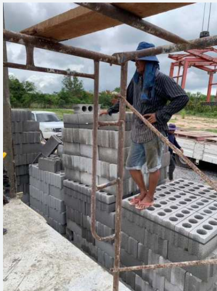
Wall construction around the structural frame.
