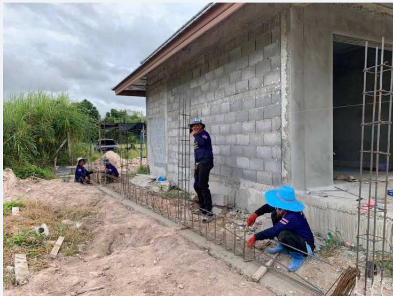
Progress of blockwork and external wall formation.
