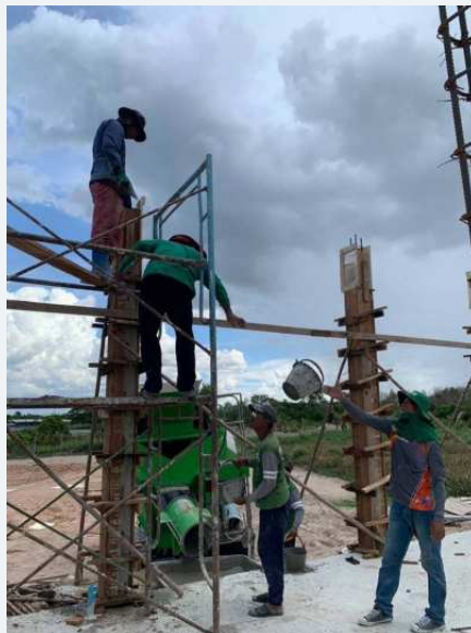
Column preparation and related structural activities.
