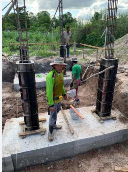
Reinforcement detailing and formwork preparation.
