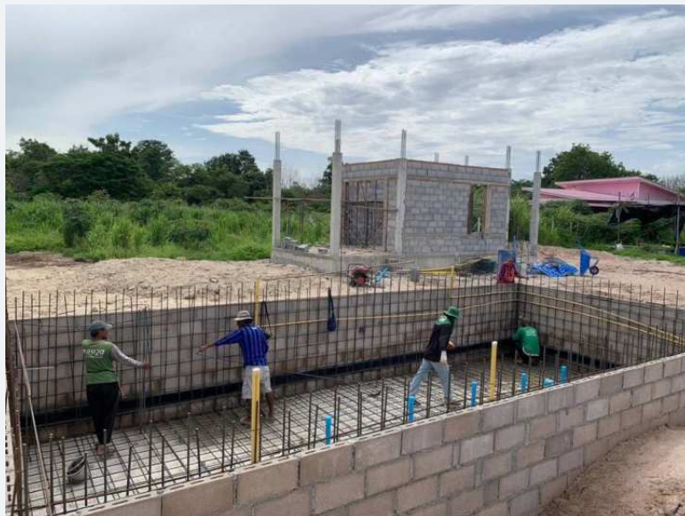
Slab formation and concrete finishing activities.
