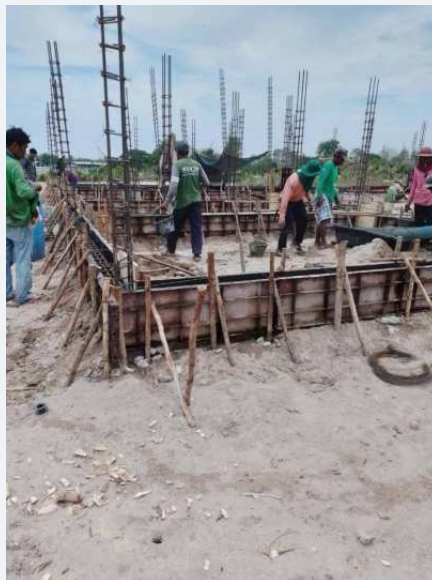
Steel reinforcement before subsequent concrete works.
