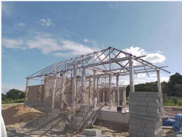
Overall view of the building during construction.
