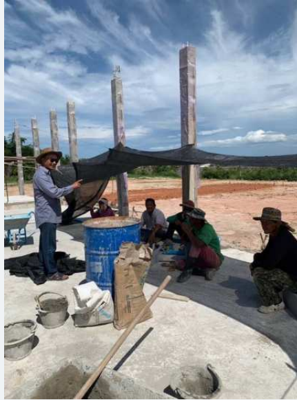
Reinforcement detailing and formwork preparation.
