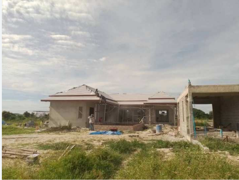
Overall view of the building during construction.
