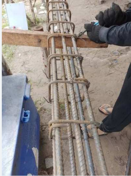
Steel reinforcement before subsequent concrete works.
