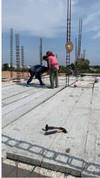
Placement and arrangement of reinforcing steel.
