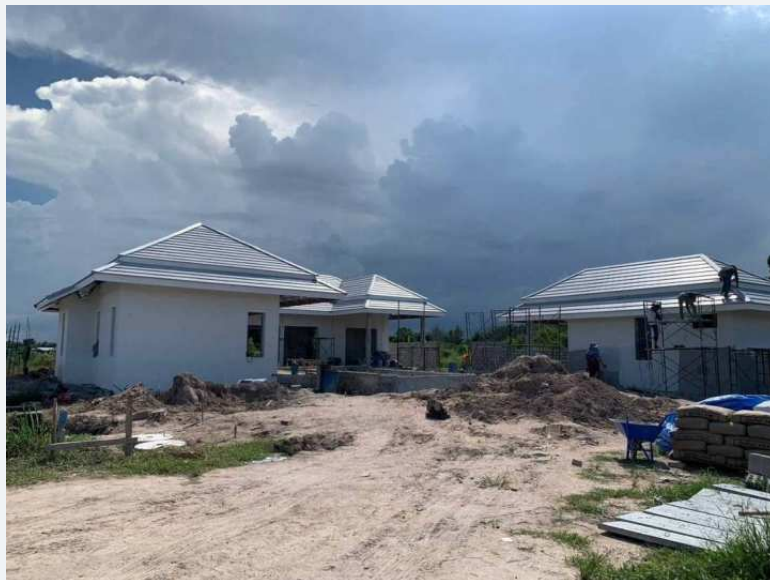
Overall view of the building during construction.
